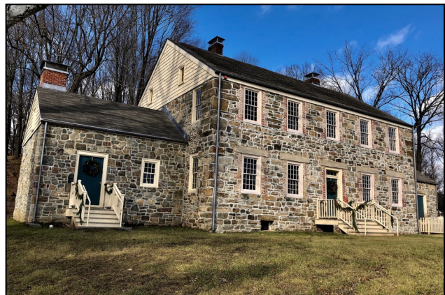
The Ford-Faesch House, located at 629 Mount Hope Road, featuring the reconstructed West Wing on the left.
